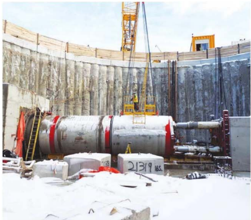
Figure 10. Microtunnel Setup for the HLI Extension in the Screen Building Shaft.
