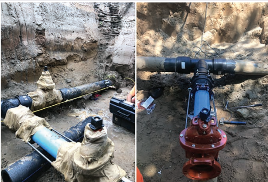
Figure 3. Different Fittings Electrofused to the HDPE Watermain
